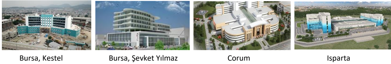
Figure 5: Monitoring of City Hospitals with Seismic Isolators
