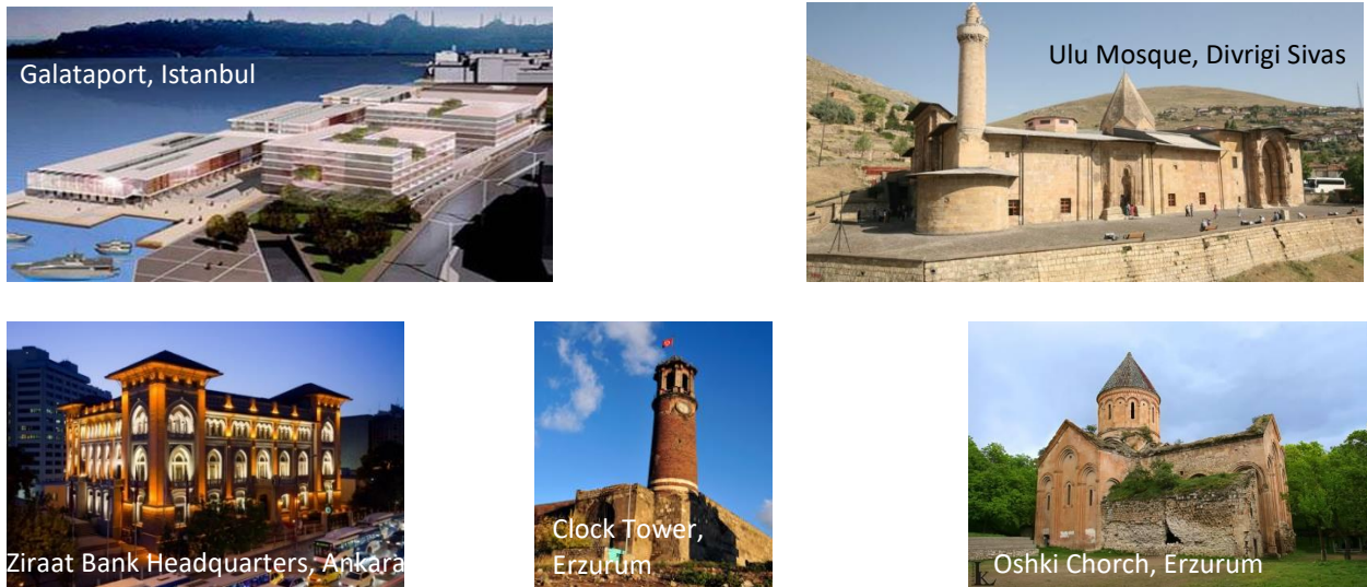
Figure 6: Extensive Monitoring Practices of Historical Structures
